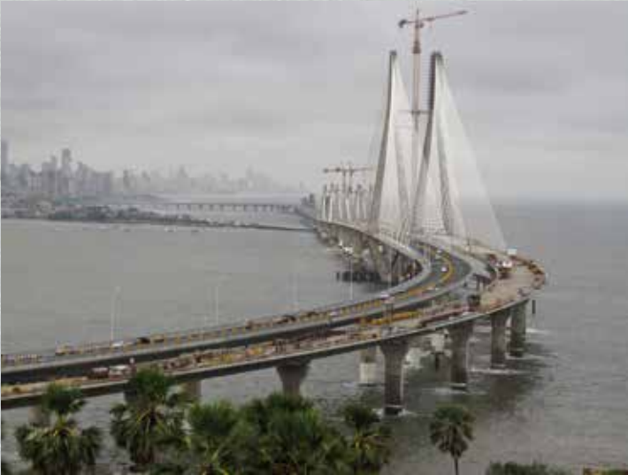
The Bandra-Worli Sea Link in western India connects downtown Mumbai to the suburbs. The pillars of the bridge, with concrete provided by UltraTech, are set in the Arabian Sea.
