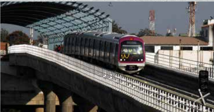
The Bangalore Metro rail project has used .79 lac MT of UltraTech cement in the first phase of the project.
